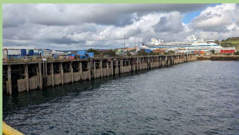
Photograph of existing causeway, taken south-east of the causeway, facing north-west
